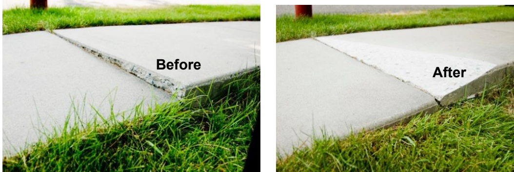
Figure 7: Precision Sidewalk Safety Work Example
