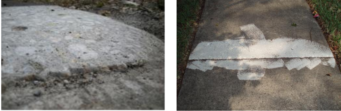
Figure 8: Typical Results from a Grinder
